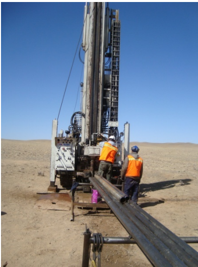
Drilling at Tsant Uul
